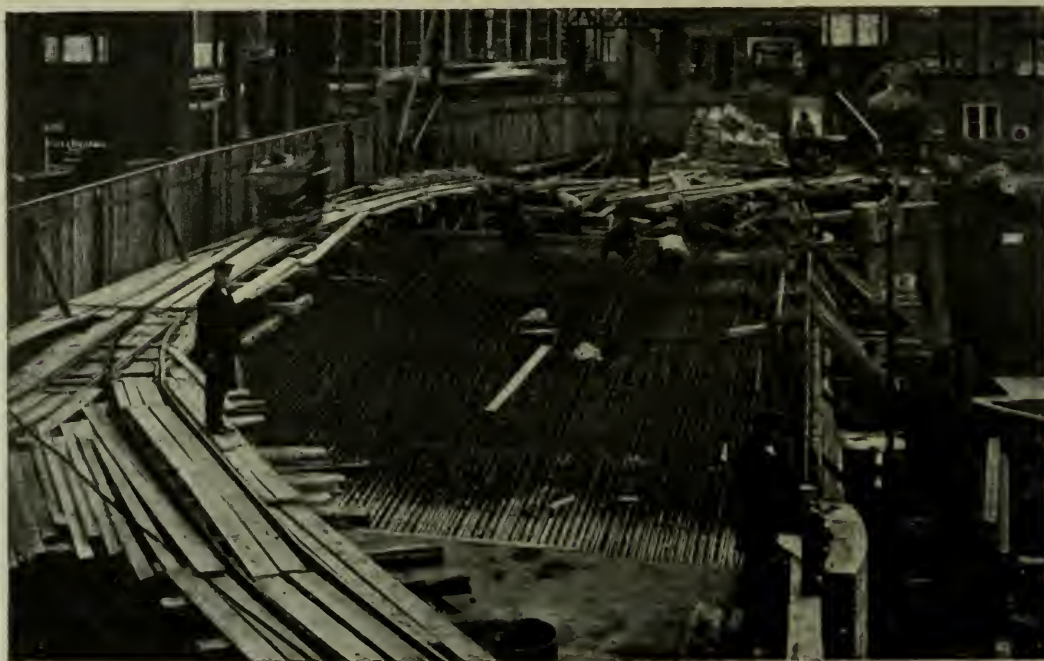
FIG. 7.—SCHAARTOR BRIDGE UNDER CONSTRUCTION.
